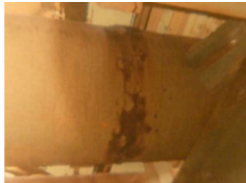
Initial condition of pipework
