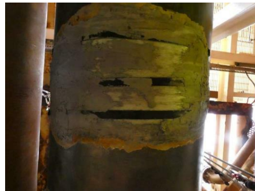
During repair application
