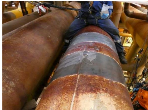
After surface preparation
