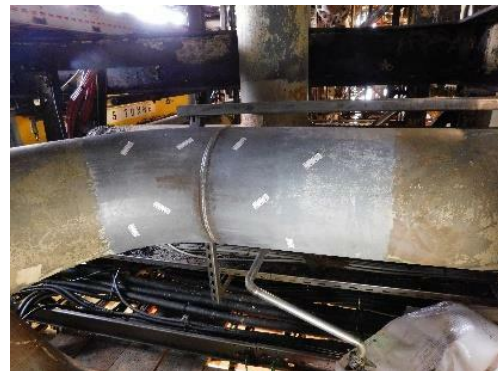
Initial condition of pipework
