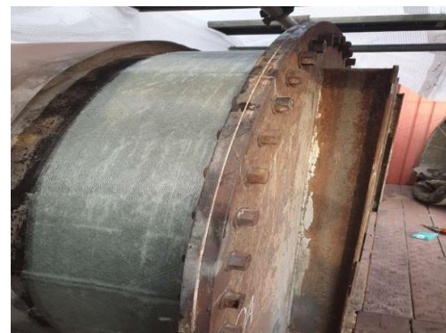
During repair application
