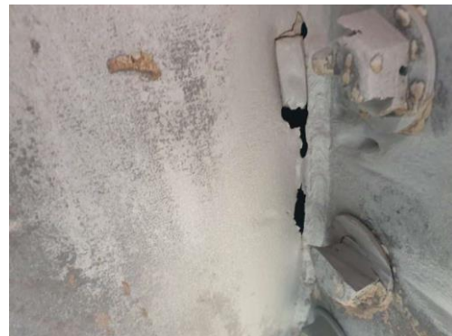
Initial status of pipework
