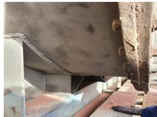
After surface preparation
