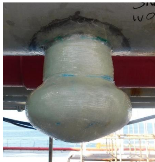
Final cured repair
