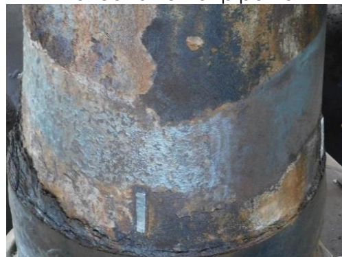
After surface preparation
