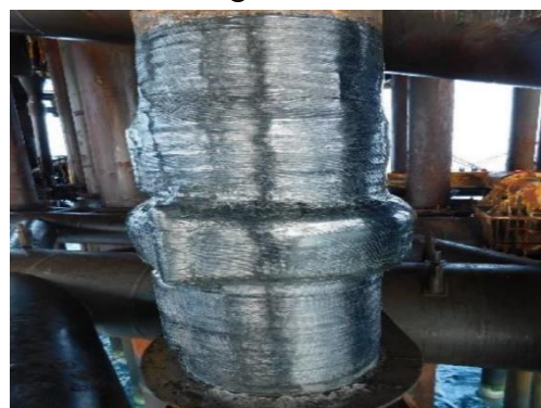
Final cured repair
