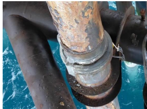
Initial condition of pipework
