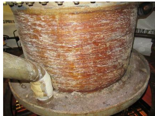
After surface preparation
