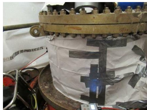
During repair application
