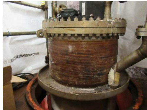
Initial condition of pipework
