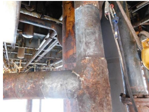
After surface preparation
